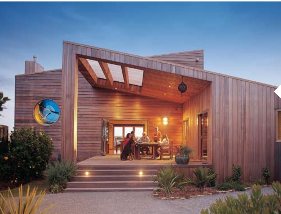
1999 MANGAWHAI HEADS This 'outdoor room' provides shelter from rain, wind and sun in most seasons and conditions. One looks through the building towards the estuary and bird reserve beyond. The design was inspired by the simple box-like shapes and mono pitch roofs of the traditional Kiwi bach. (Photography Colleen Tunicliff)
